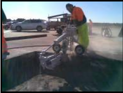
New Minnich Drill in action
