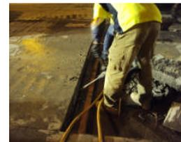
joint using 16mm drill bits on a two gang Minnich drill.
