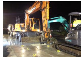
The existing lean mix was then swept free of all foreign materials and debris and inspected by both managerial staff and the client representative. Any cracks in the existing lean mix were noted on the relevant Inspection Test Plan (ITP).
