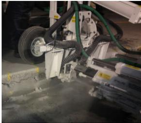
Faces of all adjacent slabs then received a coat of rapid setting paintable emulsion after which each hole was doweled using a 900mm long, R12 bar, chemset at a depth of 300mm and a 450mm long galvanized N32 dowel chemset at a depth of 225mm. Exposed N32 dowels were then also painted with the same material as the faces of all adjacent slabs.
