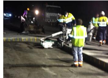
A second *Minnich Drill*® was then used to drill 38mm diameter hole in the existing adjacent slab faces across the carriage way with 3 dowels at each end of the slab beneath the wheel path.
