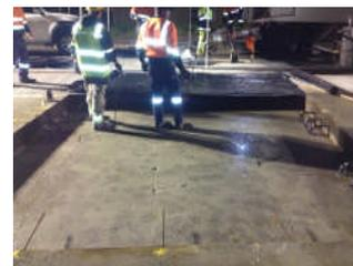
Demobilization of all plant and equipment occurred during dowel and steel installation. The concrete mixer was then parked in position ready to dispense the concrete when required.
