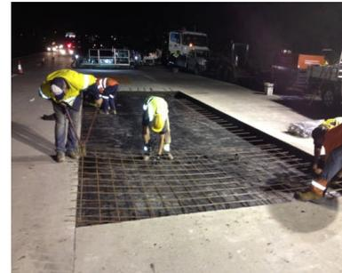
Reinforcement mesh (SL82) was then placed, lapped and tied at 250mm with a clear cover of min 50mm from all adjoining faces, N36 dowels etc.
